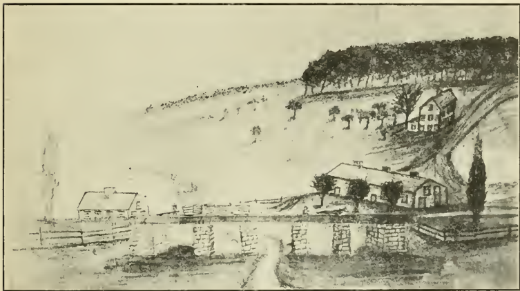
MIDDLESEX VILLAGE. AQUEDUCT, LOOKING EAST.
